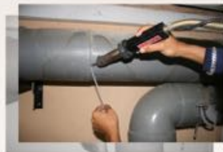
FUME EXTRACTION SYSTEM
